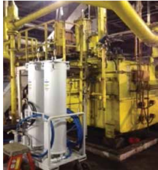
(HILCO® model 36118-53040100 installed on a customer's 2,800 GAL EHC Reservoir)
